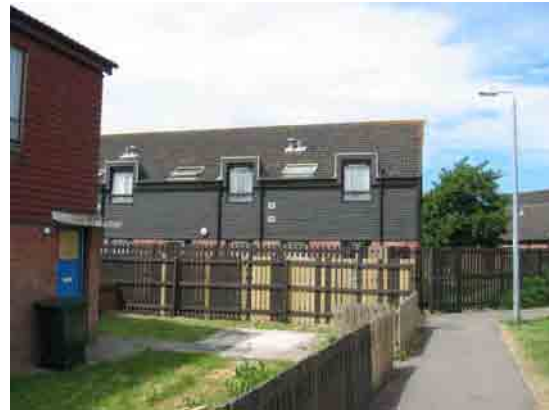
Figure 16 Pathways, high fences one side; no sight of who might be round the corner.
